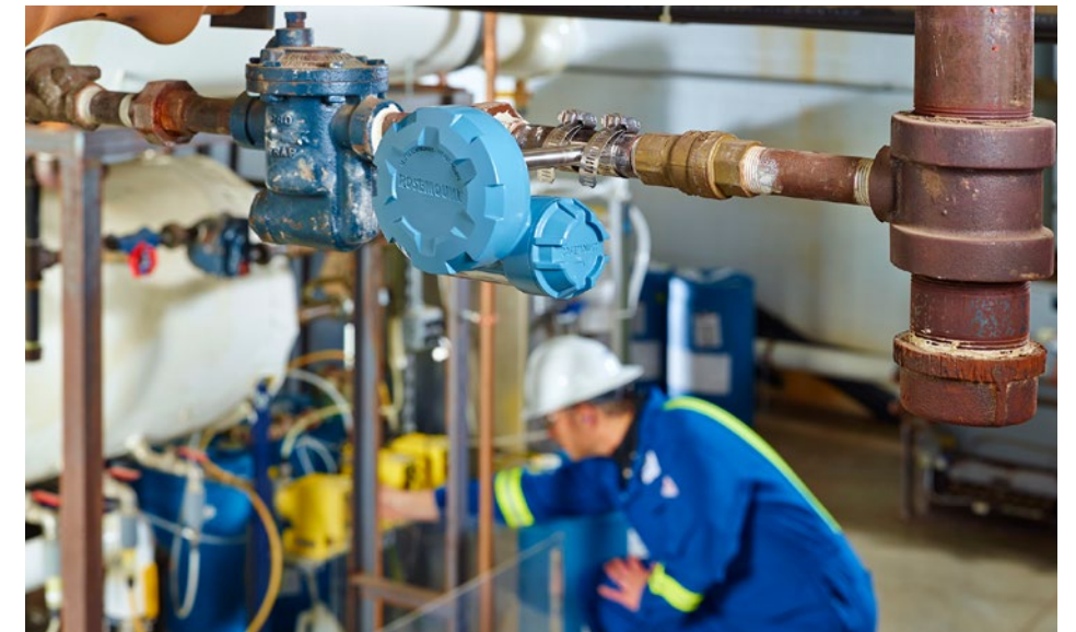
Figure 4: Emerson's Rosemount™ 708 Wireless Acoustic Transmitter provides visibility into steam trap operation and condition by analyzing ultrasonic noise signatures.
