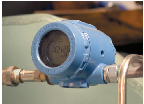
Figure 3-30 – Remote Mount Installation
