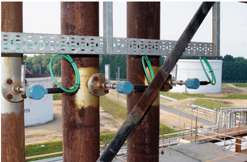
Figure 3-81 – Thermowell Installation Examples
