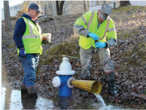
Picture 2.5: Water inspection
