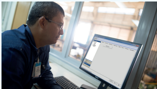
Picture 3.4b: On-line testing in the control room
