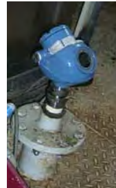
Figure 2. Installation of Rosemount 5303 Guided Wave Radar.
