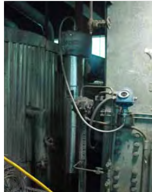
Figure 1: Rosemount 5301 with Dynamic Vapor Compensation measures reliably on boiler drum
