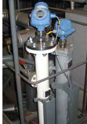
Figure 2. A second Rosemount 5301 replaces the electronic displacer.
