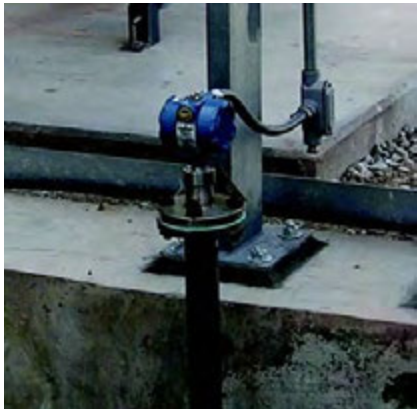
The Rosemount 3300 GWR installation only requires the loop connection and process mounting.
