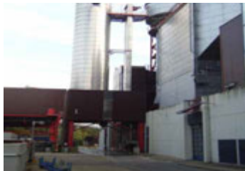
Figure 1. 60-ft (18.5 m) tall combustion salt silo at garbage incineration plant.
