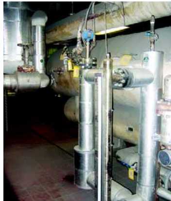
The Rosemount 3301 Guided Wave Radar Installed at the Sunbury Generation power plant.
