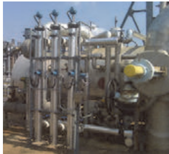
Figure 1. Feedwater heater level achieves triple redundancy with Rosemount 5300 Guided Wave Radar
