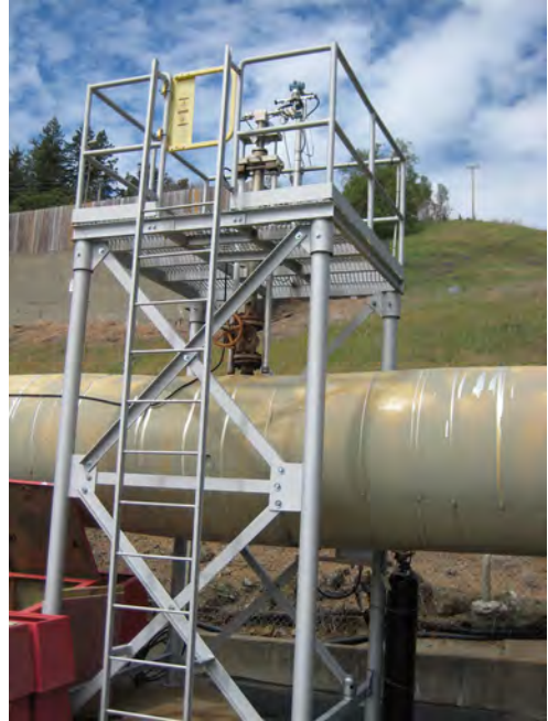
Figure 6.22: Rosemount 3051SFA Annubar Flow Meter mounted above the pipe in a geothermal steam application.
