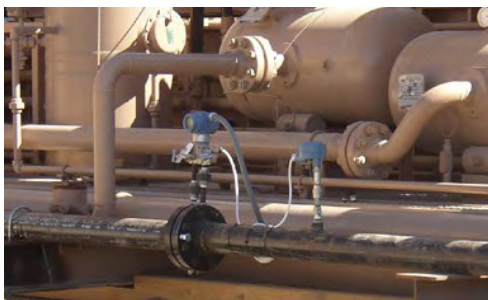
Figure 4.3: A standard orifice plate used in a natural gas application.
