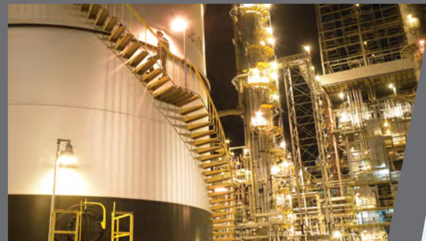
The refinery processes 250,000 bpd of crude oil. It can manufacture diesel fuel from biomass-based feedstocks.
