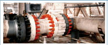
The valves' isolation and control capabilities can be combined in a single product, eliminating the usual requirement for two distinct valves, further reducing the total installed cost, weight, and footprint.
