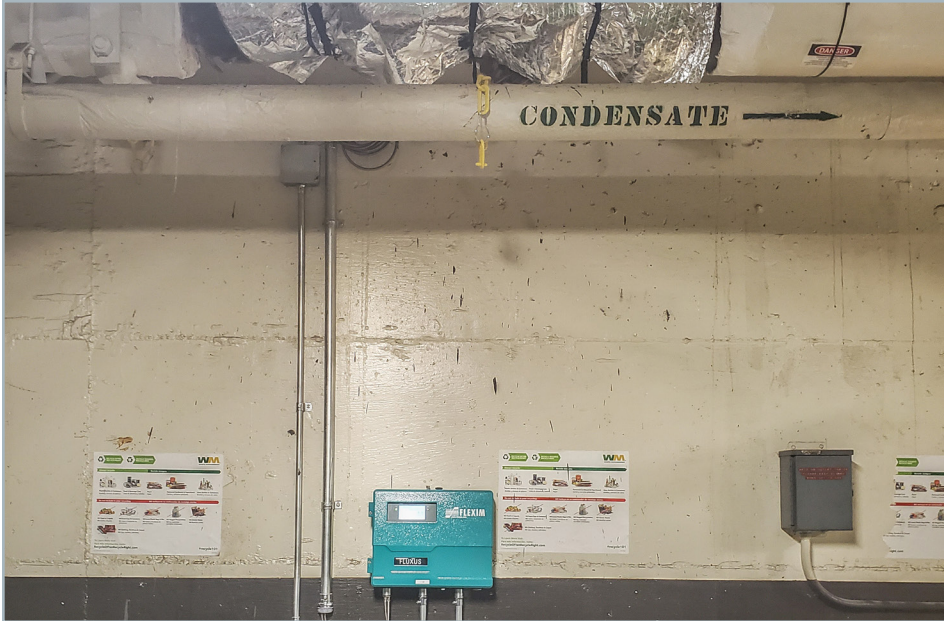
Measuring point with clamp-on ultrasonic transducers mounted in Perma-Lok rail and the stationary transmitter FLUXUS® G721 ST
