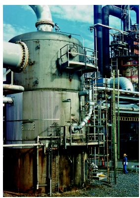
The blowdown drum is 28 ft (8.5 m) high but the required measuring range is approximately 9.8 ft (3 m). The tank can be filled to a maximum of 9.8 ft (3 m).
