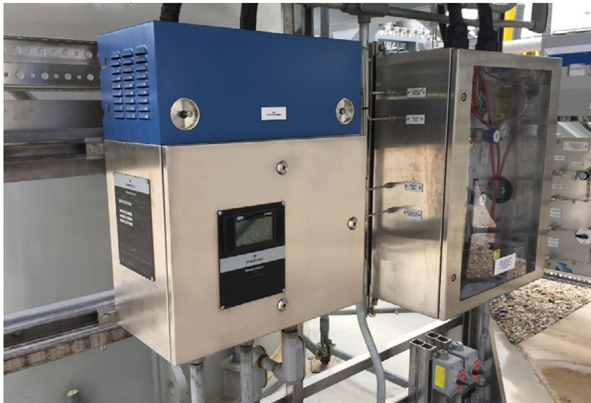
Figure 1.7: A hybrid QCL/TDL analyzer, such as Emerson's Rosemount CT5100 Continuous Gas Analyzer, can measure up to 10 gas components simultaneously in real time, from parts-per-million (ppm) to percent concentrations. It is ideal for hot/wet CEMS applications and features a purged and pressurized enclosure for hazardous areas.
