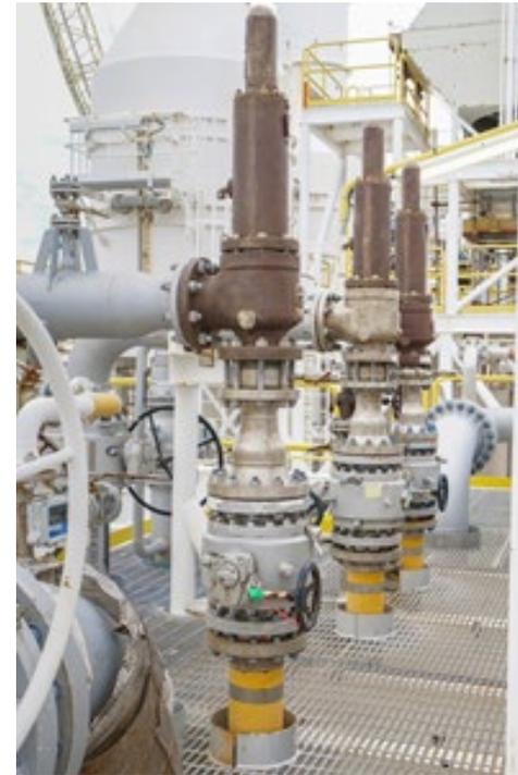
*Figure 4.2: PRVs are critical for safety, but they can create maintenance headaches. They also tend to be at the high end of piping and vessels, so access is often difficult.*
